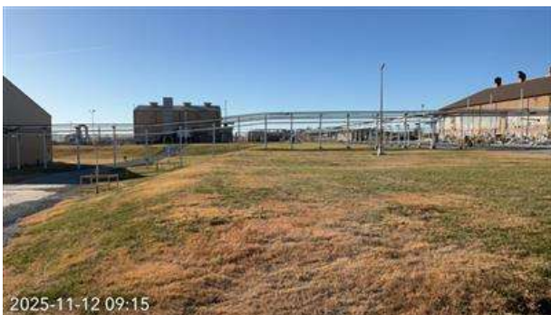
Photo 3. General view of industrial area at the Beatrice CS, photo taken facing south.
