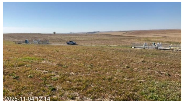
Photo 8. General view of existing Northern facilities, photo taken facing southwest.
